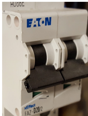
Figure G.1: Circuit breaker in the OFF position
