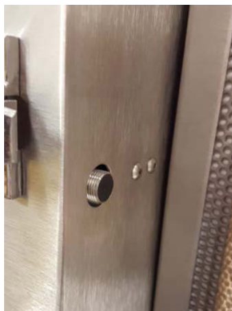
Figure G.3: RTFO door proximity switch
