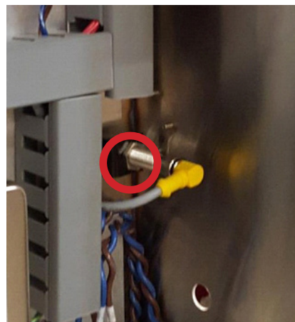
Figure G.4: Side panel removed, exposing the door proximity switch. Adjustment nut indicated in red.
